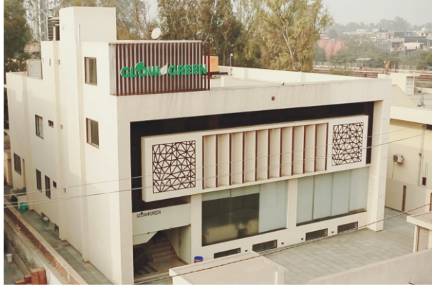
Corporate Office / R&D Centre / Production Unit
